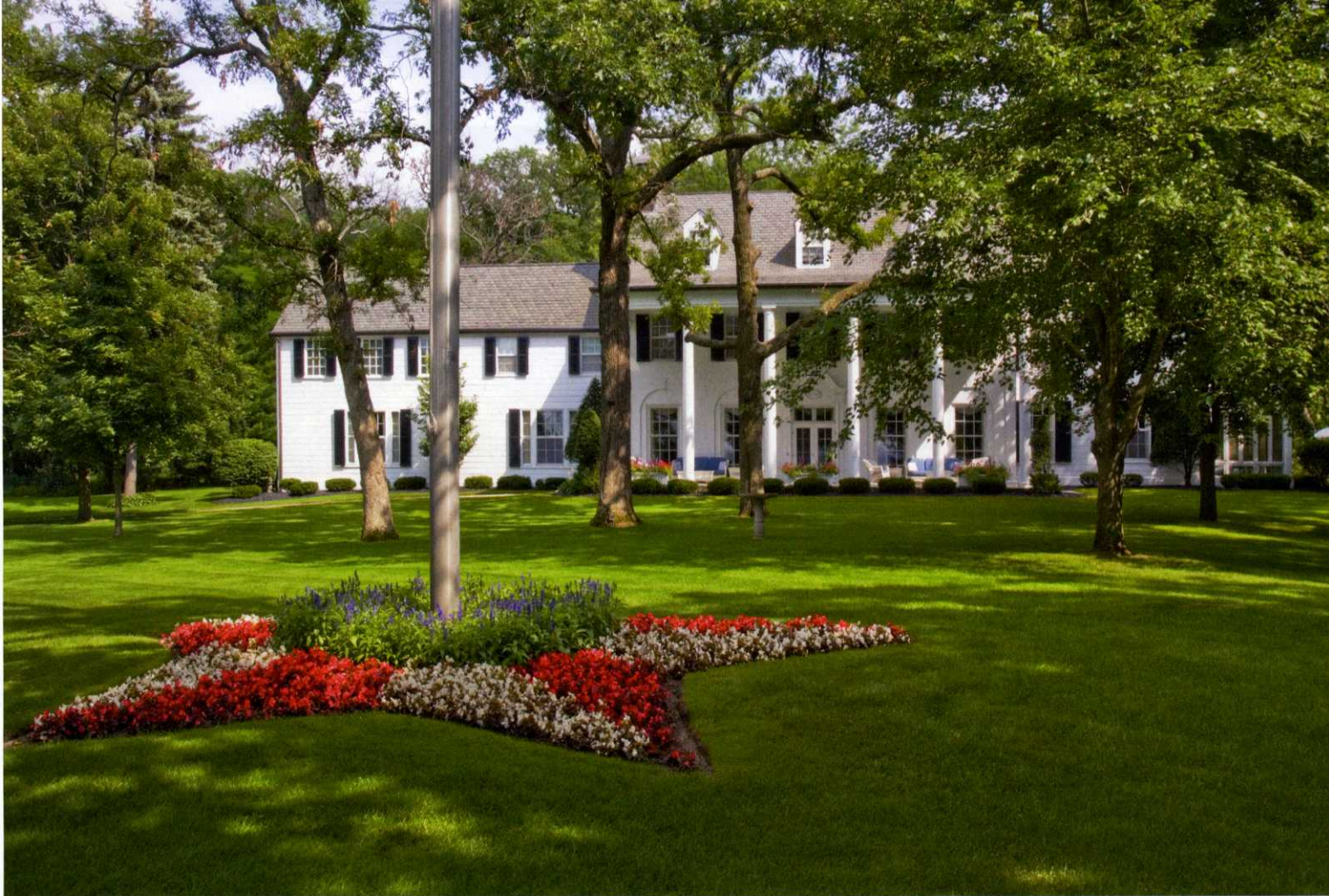
■ Designed by Howard Van Doren Shaw for Lewis Edward Myers in 1924, this sprawling Lake Geneva estate is an example of the architect's "country house" design. Dubbed "Allegheny," the home has been in the current owners' family since 1945. Myers was said to be an avid orchid grower with some 200 rare specimens on the property garnering international attention. The recent landscape renovation has put the historic home and garden back in the spotlight.
